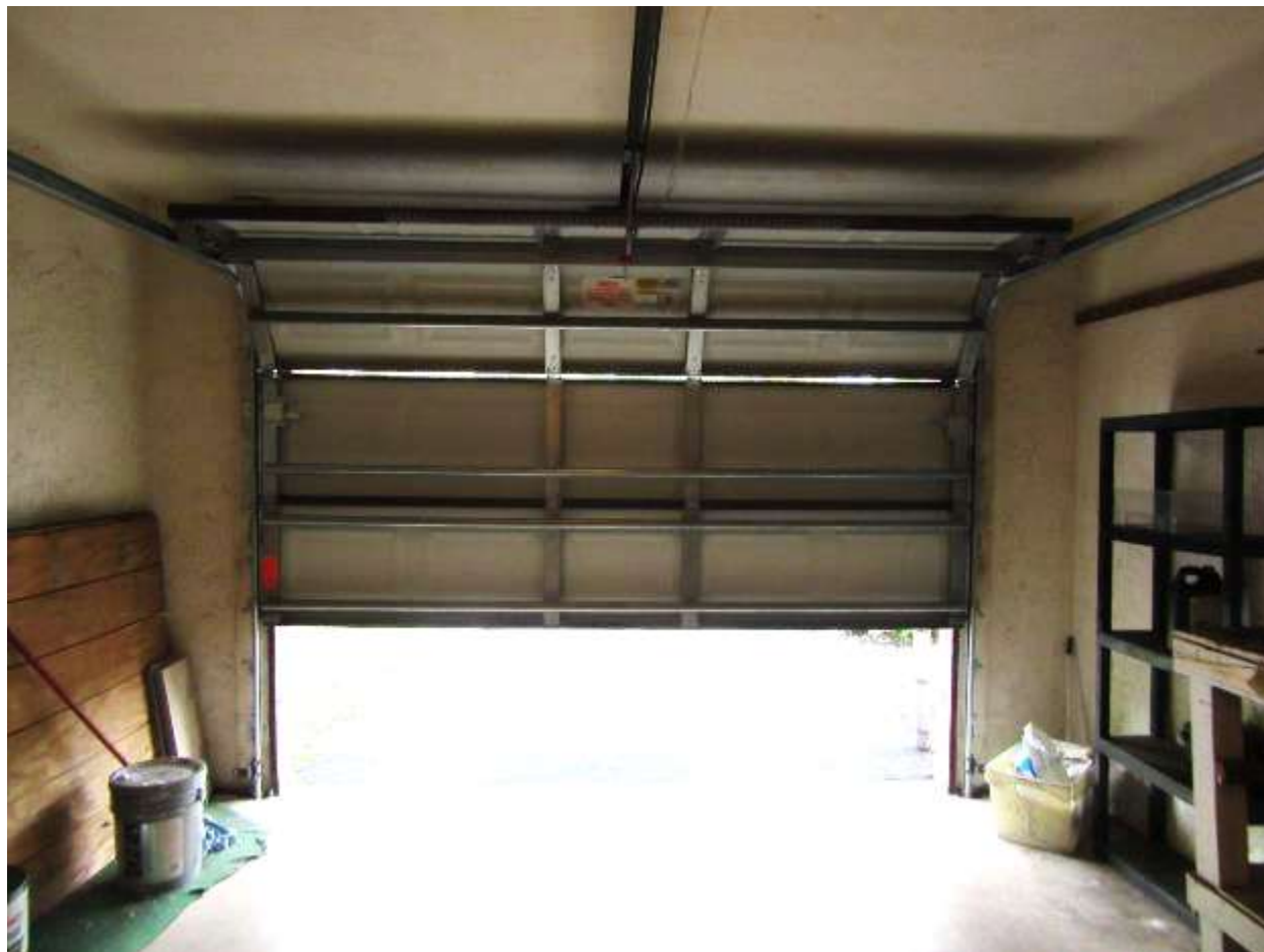
Garage door in good working condition at the time of inspection.
