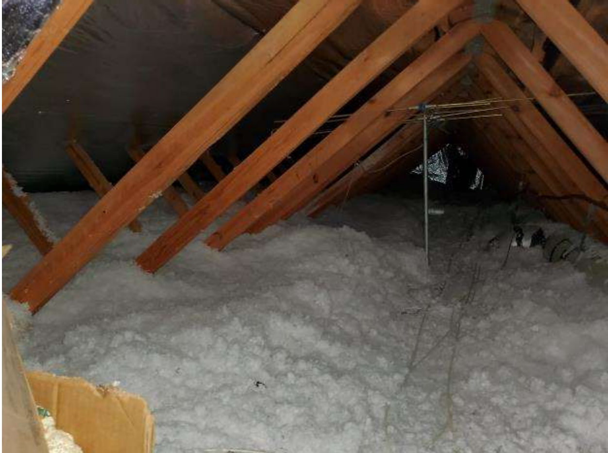
Attic space where accessible was noted properly insulated
